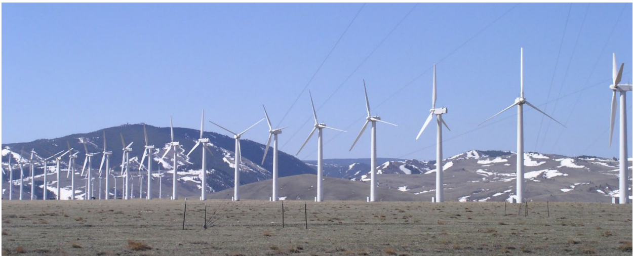
Wind farm in Wyoming on BLM-managed public lands.
