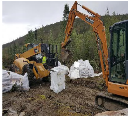
Loaders haul out solid waste debris and remove contaminated soils from the site
