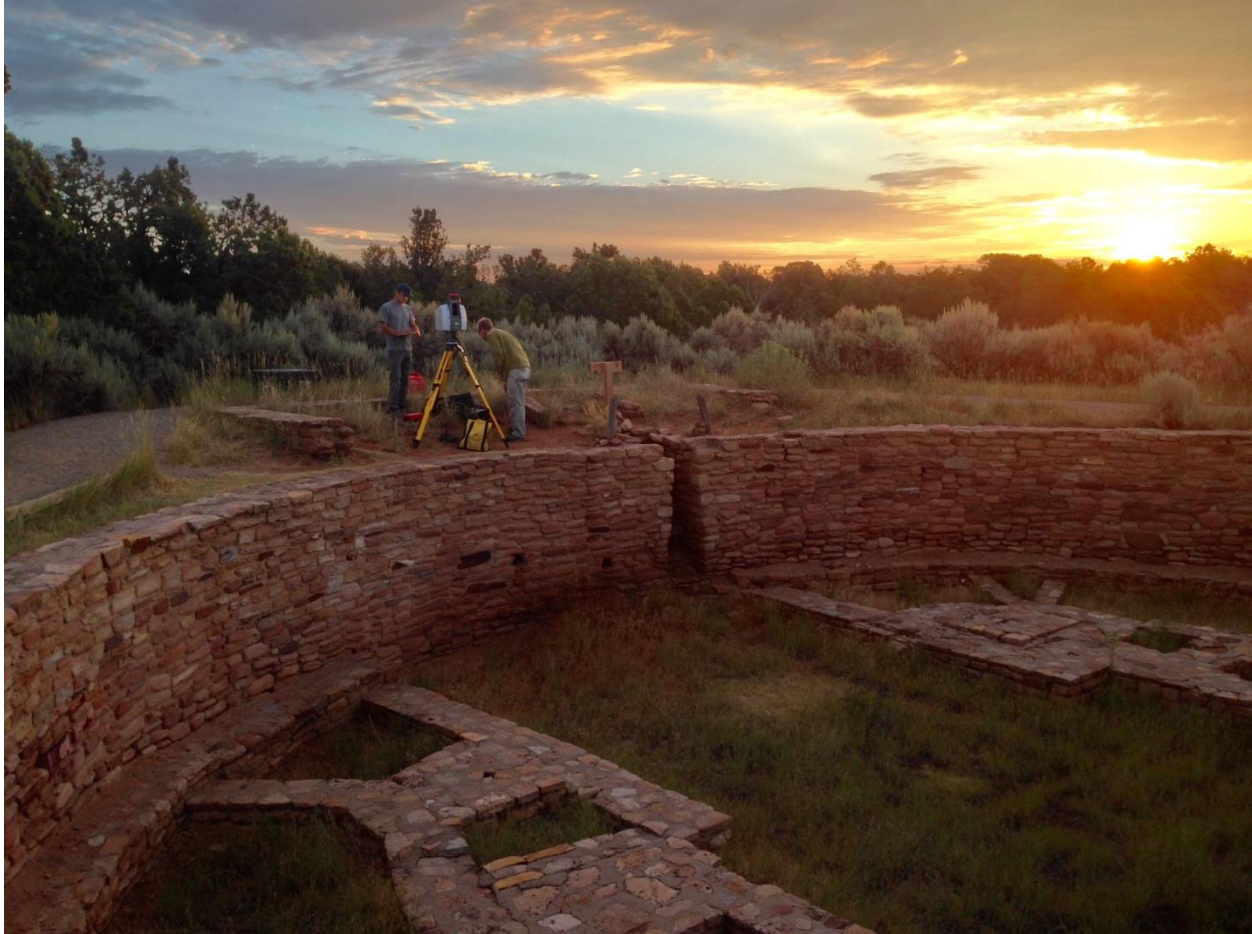
Staff and students of the University of Colorado at Denver School of Architecture and Planning's Center of Preservation Research and CANM continued work implementing the Monument's Digital Documentation Protocol at Lowry Pueblo National Historic Landmark (5MT1566), Canyons of the Ancients National Monument, Colorado.
