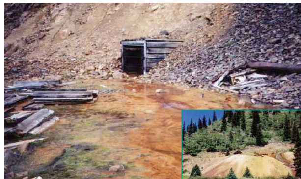
BLM can address injuries at abandoned mines through the NRDAR Process
