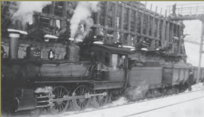
V & T locomotive #25 delivering building materials to the mill during construction. Joe Curtis Collection.
