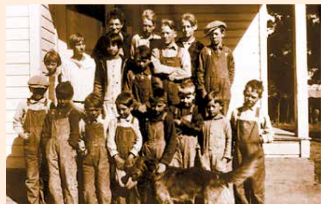
Students from the one-room Goodman Point School pose on the front steps with a favorite dog. The school is now privately owned.
