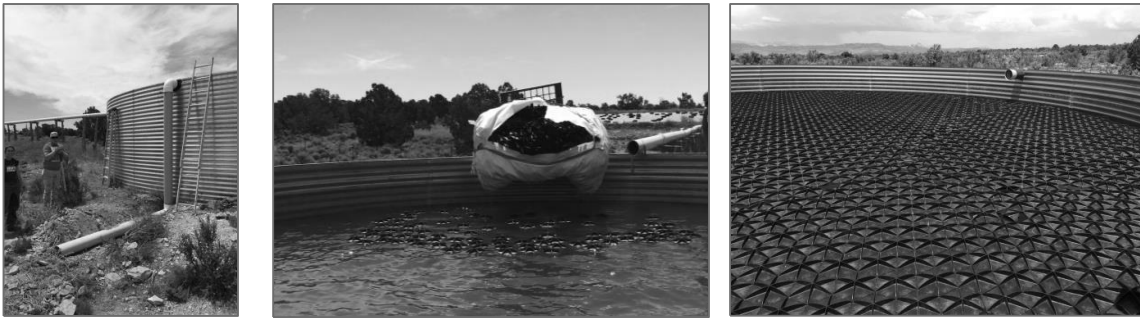
Left: Seasonal range and fire staff assist in construction of overflows. Center: Hexa-cover discs being added to a large storage tank. Right: The floating discs are beginning to interlock to form a semi-solid lid. These lids reduce evaporation by 95% and reduce wildlife mortality.
