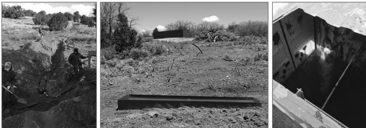
Left: Staff replacing valves on the West Clark pipeline. Center: Newly replaced wildlife drinker in foreground and water storage tank in background at Timber Mountain. Right: Rain water flowing into the new tank at Timber Mountain.
