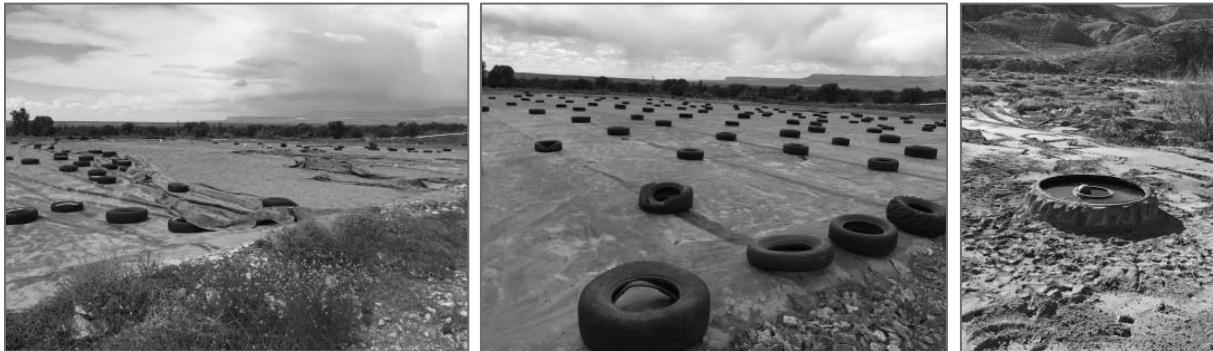
Left: Five Mile catchment apron before repair. Center: Five Mile apron after repair. Right: New tire trough replacing an old trough at Coyote Wash.
