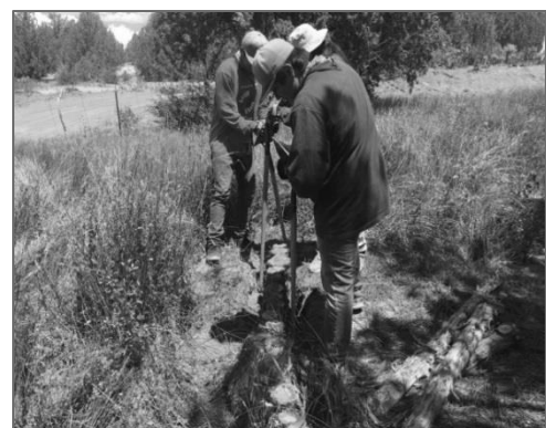
Installation of a sediment collection structure at Old Corral Spring to control erosion and rebuild the system.
