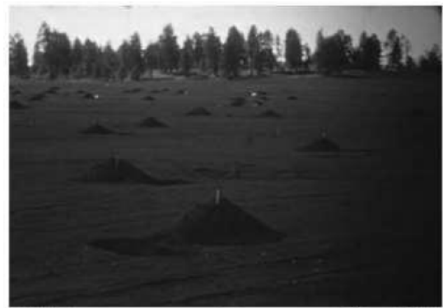
The moon's Mare Tranquillitatis is an ancient plain of volcanic rock pocked with craters and coated with fine dust. In the 1960s, engineers and scientists in the U.S. Geological Survey's Astrogeology Branch reproduced a 10-acre swath of Mare Tranquillitatis in Corder Lake, a volcanic crater field northeast of Flagstaff, Arizona, for use in Apollo astronaut training and lunar vehicle and equipment testing. This video shows how they marked out crater locations, planted explosives, and set them off in three waves, excavating hundreds of craters up to 10 meters wide.
