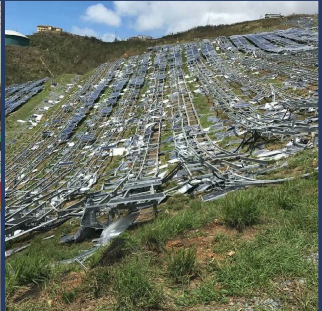
Damage to solar panel fields
