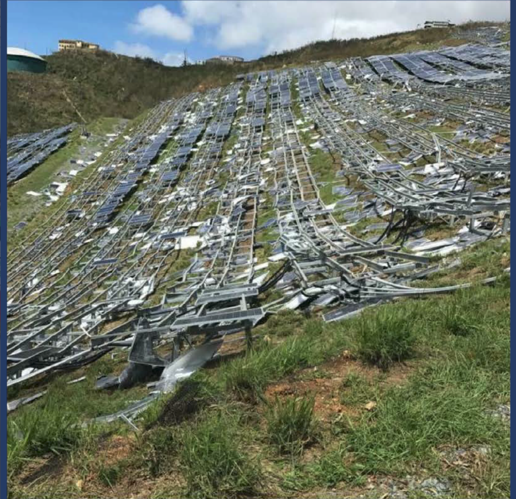
Damage to solar panel fields
