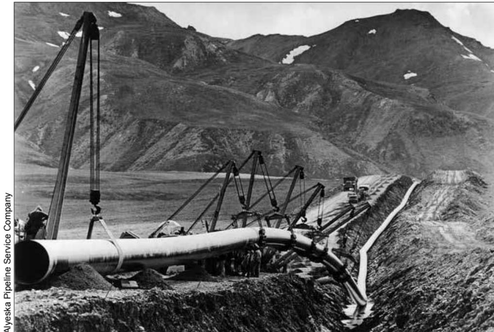
A section of the Trans-Alaska pipeline is lowered into a ditch in the Brooks Range in August of 1976, about 175 miles south of Prudhoe Bay.
