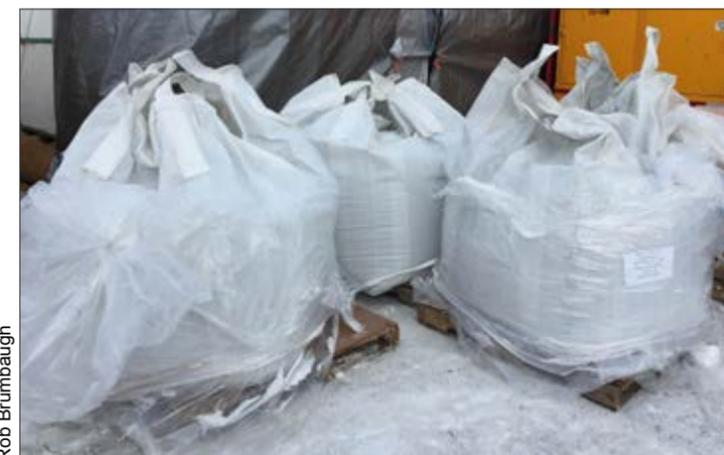
The contractor used large bags of cement to plug the wells. It took about 25 bags to plug these three wells.
