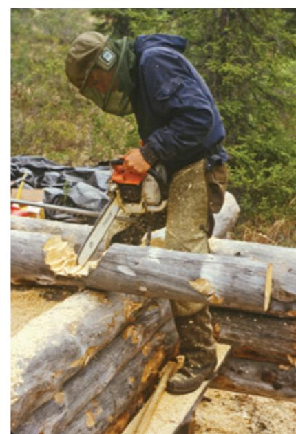
Notching logs with chainsaw.
