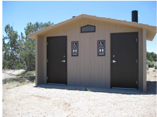
Double vault toilet at Rocky Peak Campground
