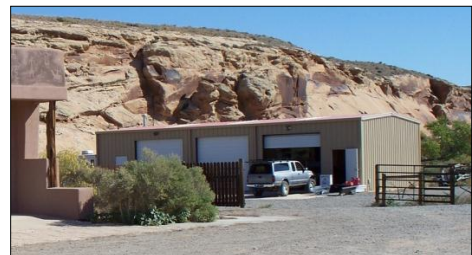
The solar-powered ranger station at Sand Island (left) is a visitor contact station, and along with the river equipment warehouse (below), serves as the operational base for BLM San Juan River rangers.
