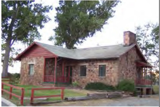
This structure is located at the Stewart Indian School in Carson City. It was probably constructed in the late 1920s - early 1930s, and is similar to several rustic style Zephyr Cove residences. Maplec
