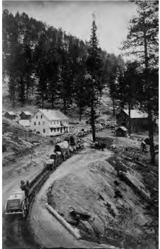
Special Collections, University of Nevada - Reno Library Swift's Station on the King Canyon Road, about 2 miles east of Spooner Summit. Note the triple wagon, and the smaller wagon waiting at the pullout.
