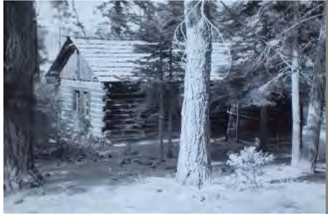
Railroad tie construction.
