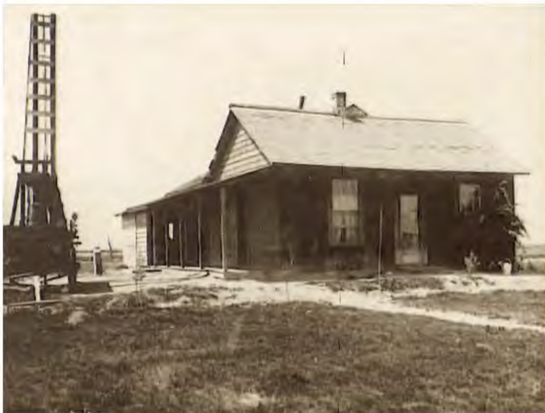
Photo 6. Well drilling beside the Munson home, 1911. Courtesy of Leonard R. Munson.
