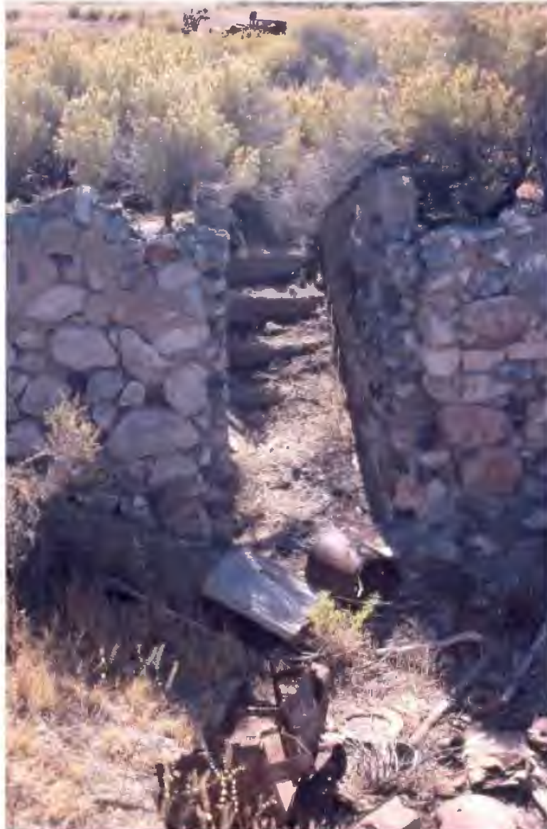
Photo 11. Remains of Thomas J. Sweeney's root cellar, with rock walls and cement steps, located behind the family's house. Taken by the author, 2005.
