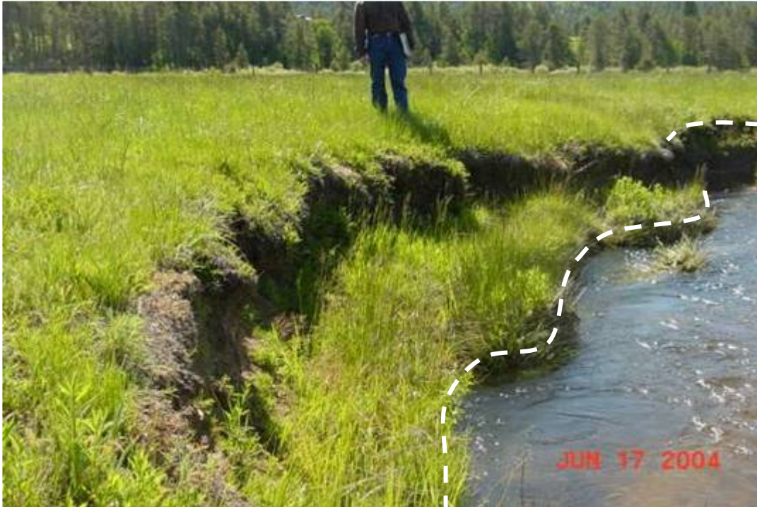
Figure 11 —this is a false bank (FB) and is stable.
