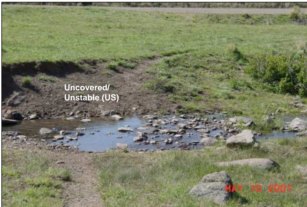
Figure 24 —highly compacted areas such as this livestock trail and slough is directly entering the stream is classified as uncovered/unstable (UU).
