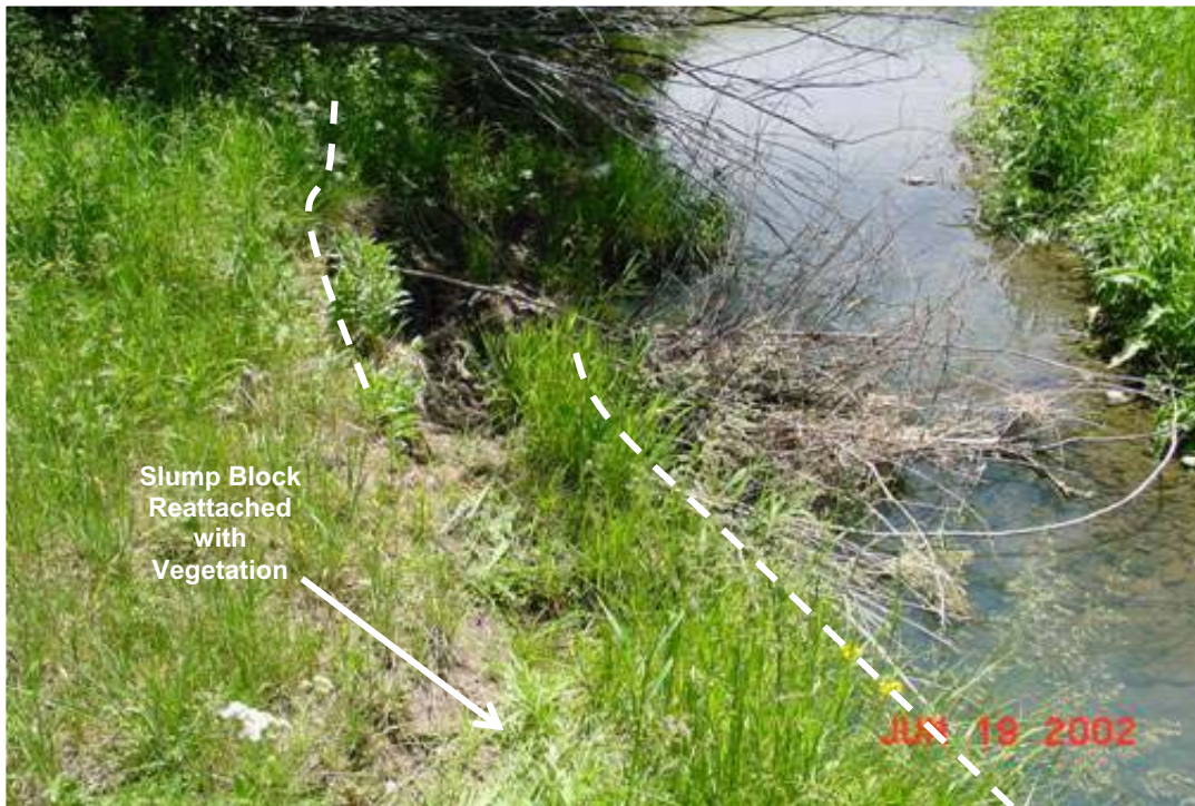
Figure 27 —vegetation attaching slump feature to the streambank creating a new floodplain. This is sometimes referred to as a “false bank.”
