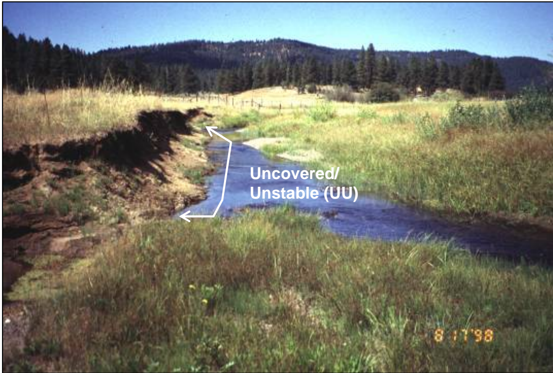
Figure 25 —the streambank is not covered with vegetation, rock, or wood. It has a bank angle of more than 10 degrees from vertical with no terrace to capture the sediment and thus the sediment enters directly into the stream making it uncovered/unstable (UU).
