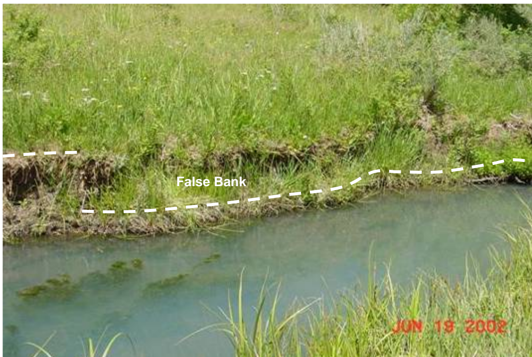
Figure 10 —false banks are slump features that is reattached and with deep-rooted vegetative cover and is stable.
