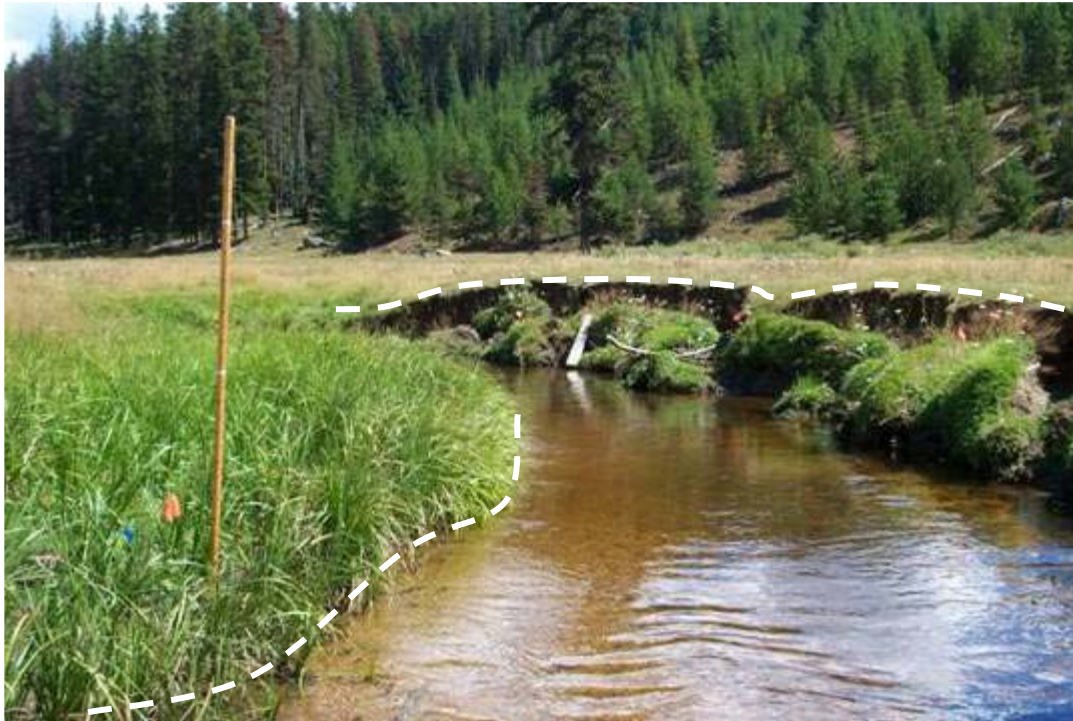
Figure 25 —slump blocks along the far streambank are not attached by vegetation to the terrace wall. Photo - PIBO, U.S. Forest Service
