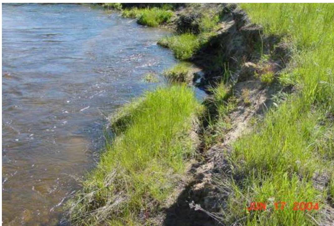
Figure 6 —the slump bank is still attached to the bank above the scour line and is covered/unstable (CU) (see Illustration 4)
