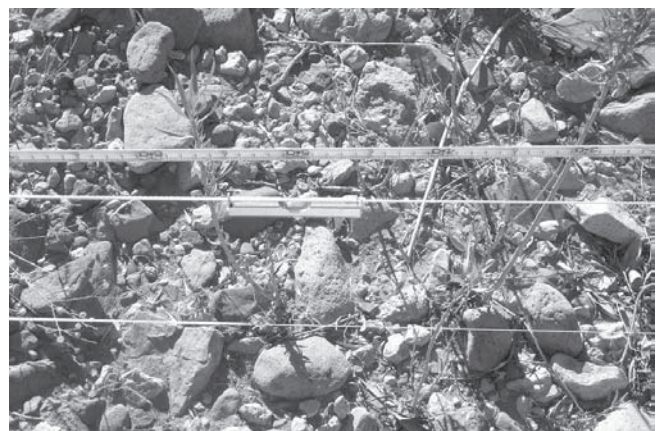
Figure 14.2. Level the string across the channel.
