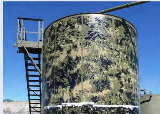
Affix the stencil, and apply the second color.
