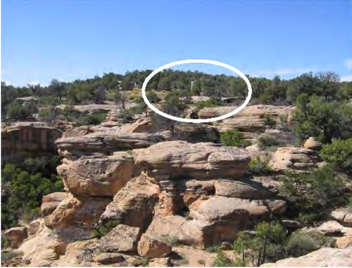
While a slightly darker shade may have been better for this tank, this single-color application successfully minimizes its visual impact.
