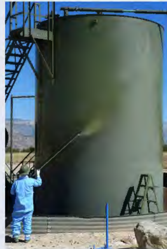
Apply the base coat.
