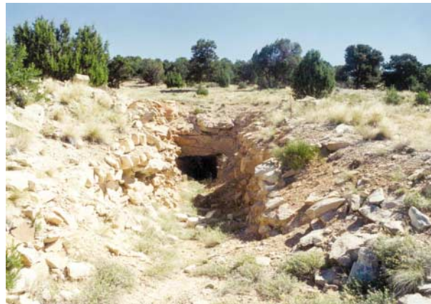
Figure 2. A typical trench portal leading to a uranium mine in western Colorado.
