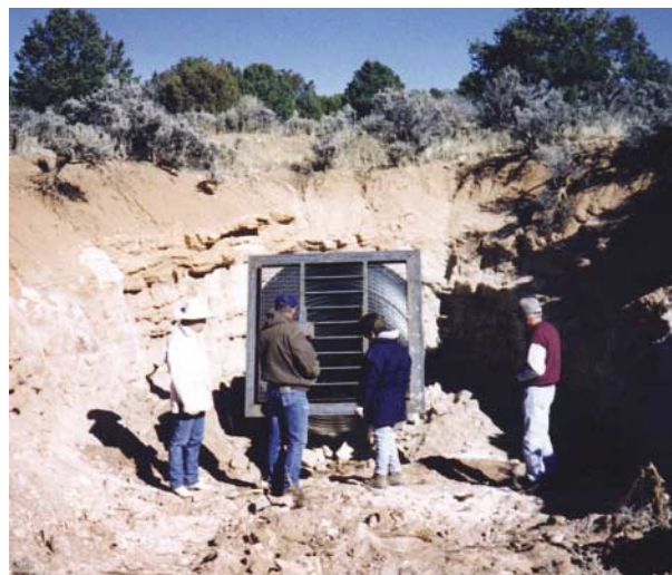
Figure 3. A culvert gate prior to backfilling the trench.
