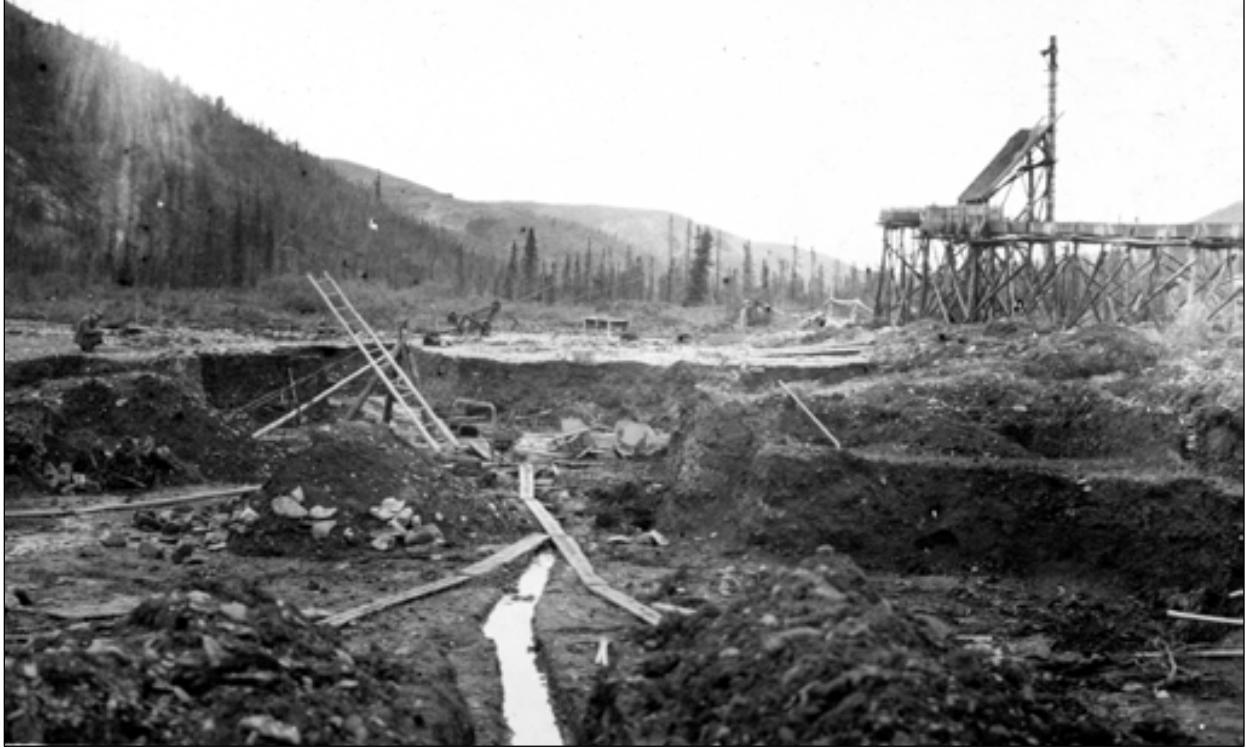
Figure 26. Historic placer mining operation on Flat Creek in 1913; miners are removing shallow overburden by hand methods to expose gold-bearing gravel near bedrock (photo courtesy of the U.S. Geological Survey)
