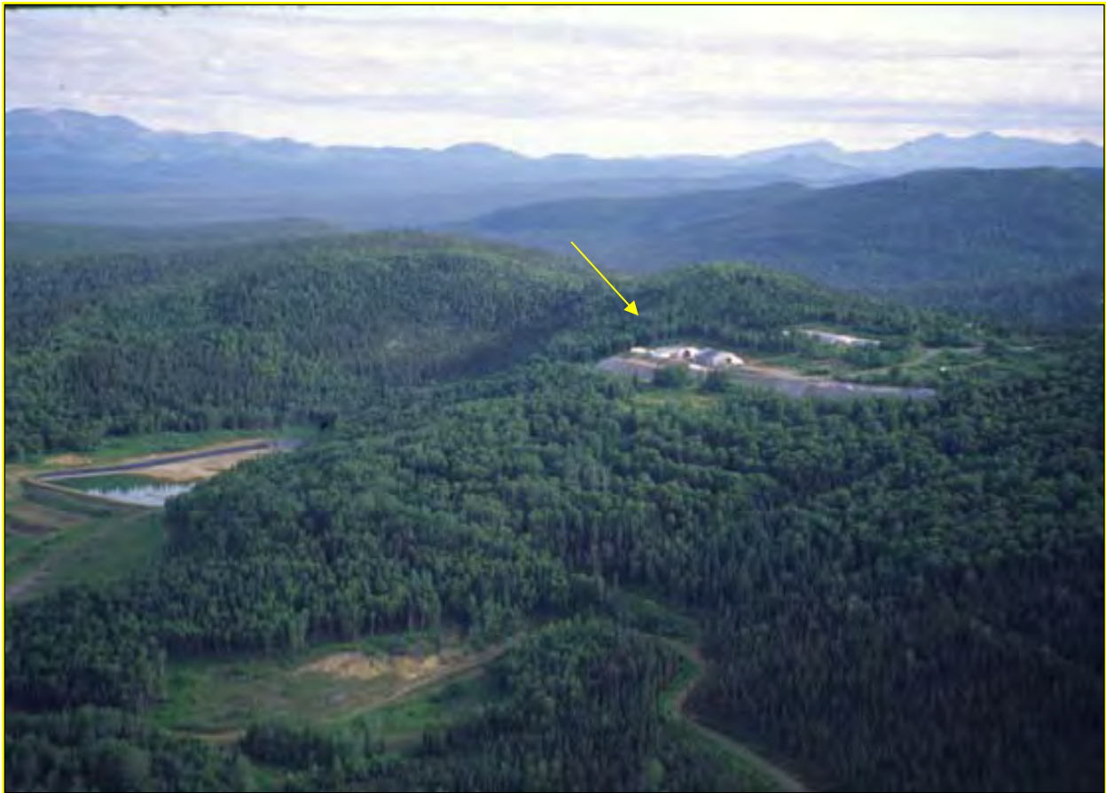
Figure 17. Nixon Fork Mine surface facilities including camp and milling complex (arrow); view to the northeast
