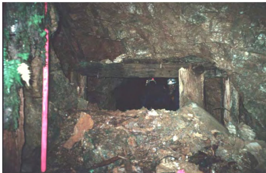
Photo 15. Geologists working inside the Hattie adit portal. Photo by P. Bittenbender.
