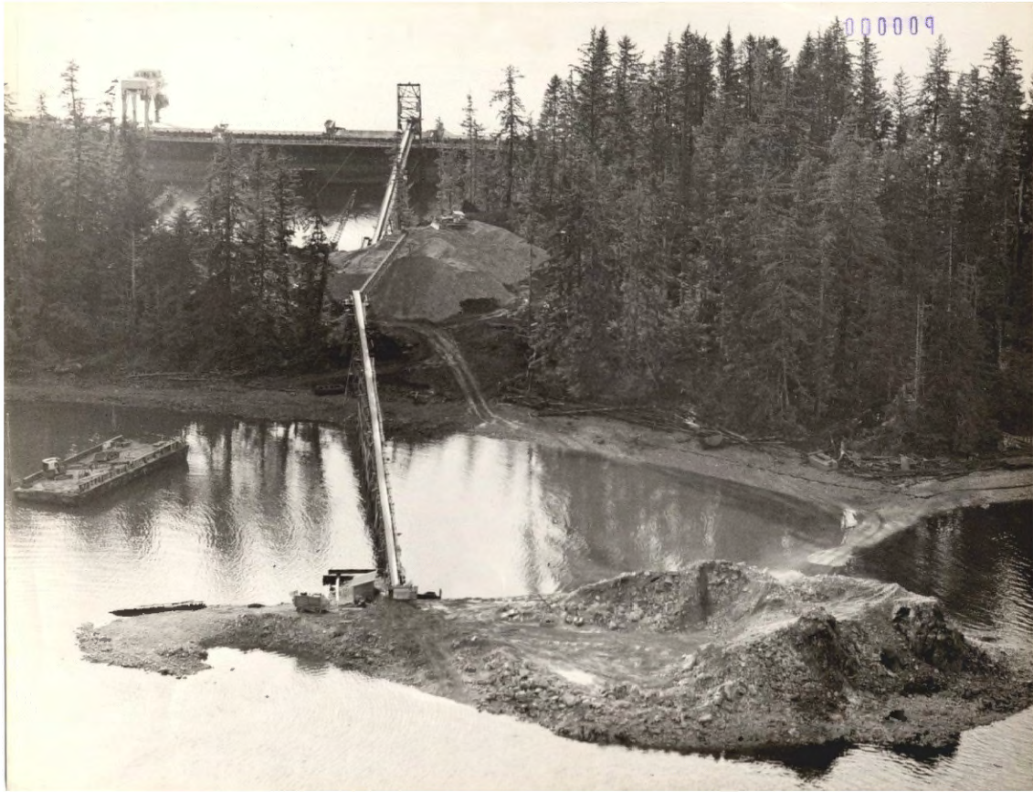
Photo 12. Conveyors loading barite on a barge at the Castle Island Mine. This photograph was taken in about 1968 when barite was still being mined from the surface. Photo from BLM archive.
