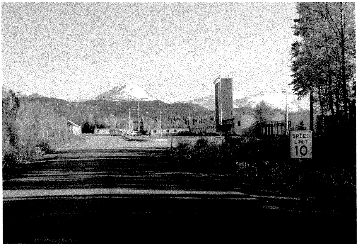
Figure 28. Developed area, Campbell Tract Facility.
