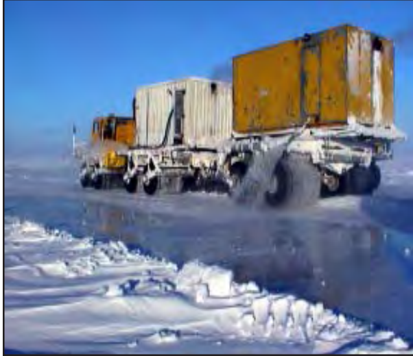
Figure 7. Water added to ice road layer.
