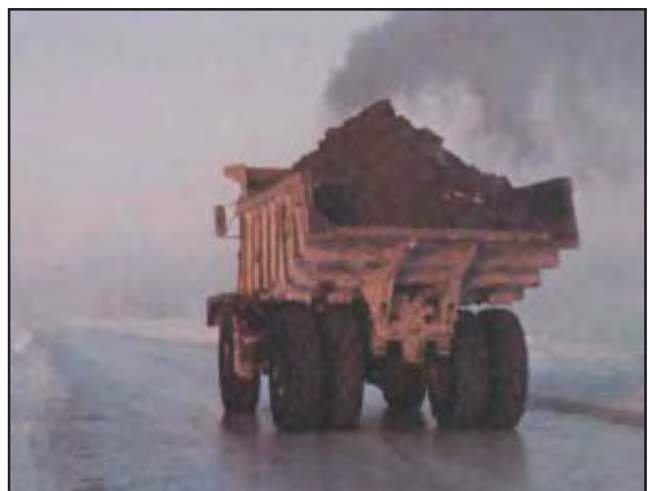
Figure 6. Gravel was hauled each day in two 10-hour shifts.
