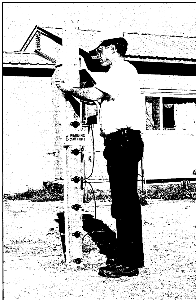
Figure 4. Electric fence gate at BLM's Seven Mile Administration Site.
