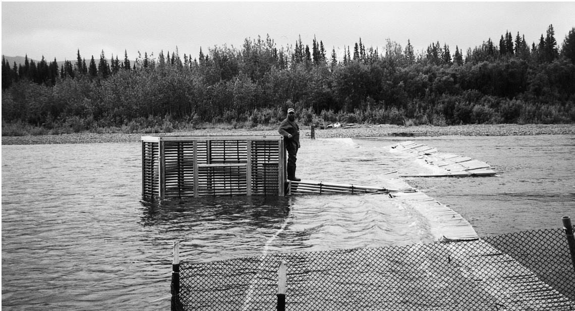
FIGURE 2 Installed weir and trap.
