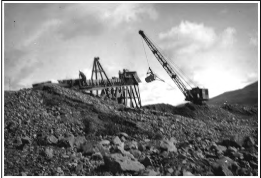
Figure 57. Barnett Photograph #55: Ed Olson's dragline mining the old Gugg Dredge tailings near the Matheson Camp, 1935.
