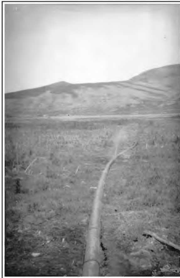
Figure 30. Barnett Photograph #28: Pipeline from the Riley Ditch, 1935.
