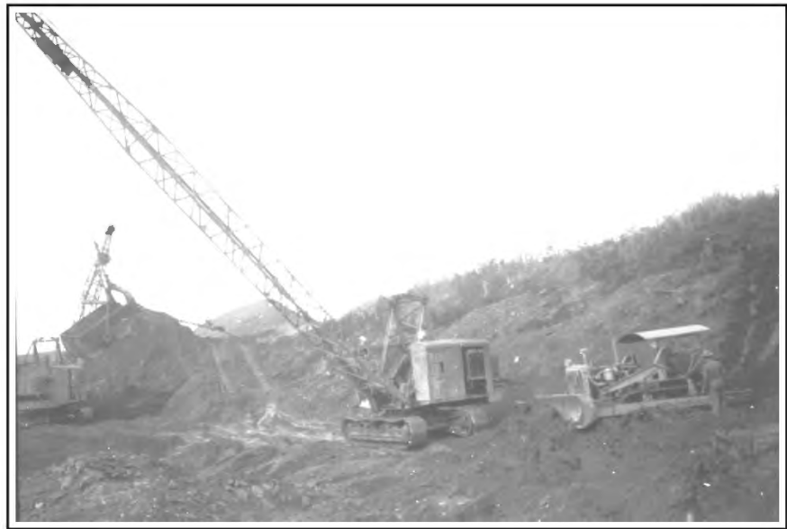
Figure 43. Barnett Photograph #41: Dragline and bulldozer operating on Happy Creek, 1937.
