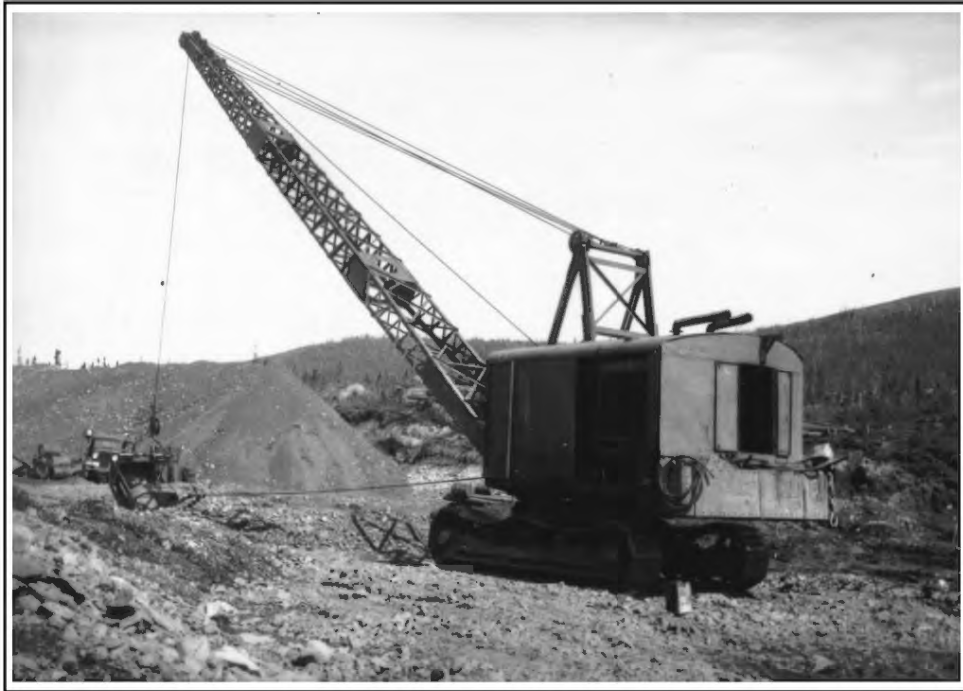
Figure 33. Barnett Photograph #31. The Uotila and Ogriz dragline operation on Slate Creek, 1937.
