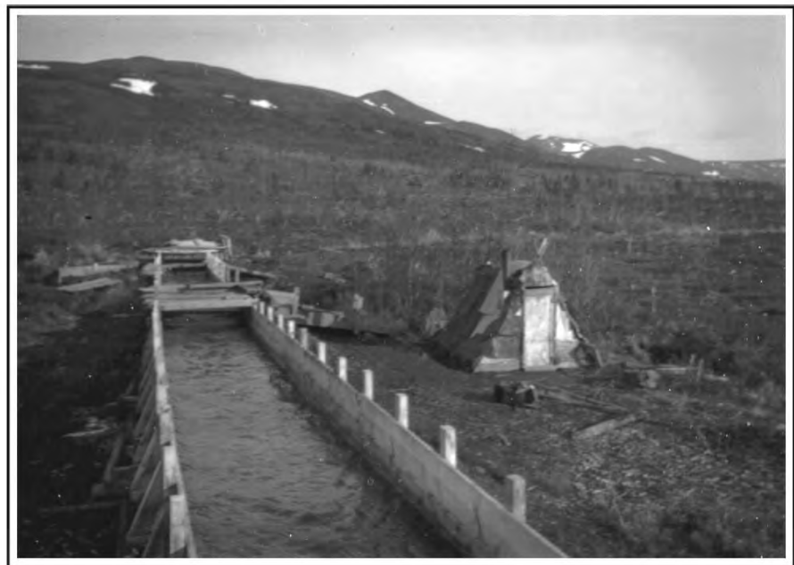
Figure 16. Barnett Photograph #14: Flat Creek Ditch and ditch maintenance shack.
