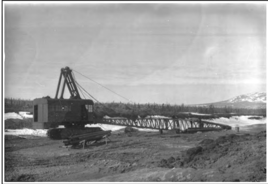
Figure 23. Barnett Photograph #23: Pete Jensen's dragline on Willow Creek.
