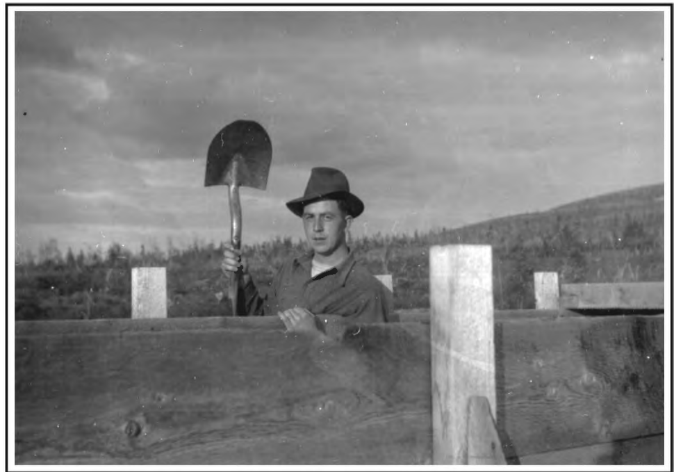
Figure 14. Barnett Photograph #12: Jack Davidson working on the Flat Creek Ditch, 1936.
