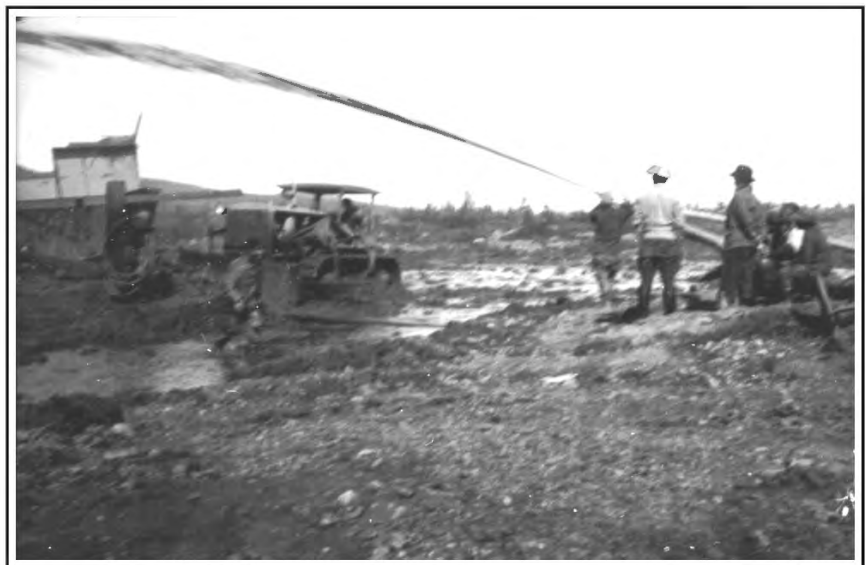
Figure 46. Barnett Photograph #44: An hydraulic mining operation using a tractor on an unidentified creek.
