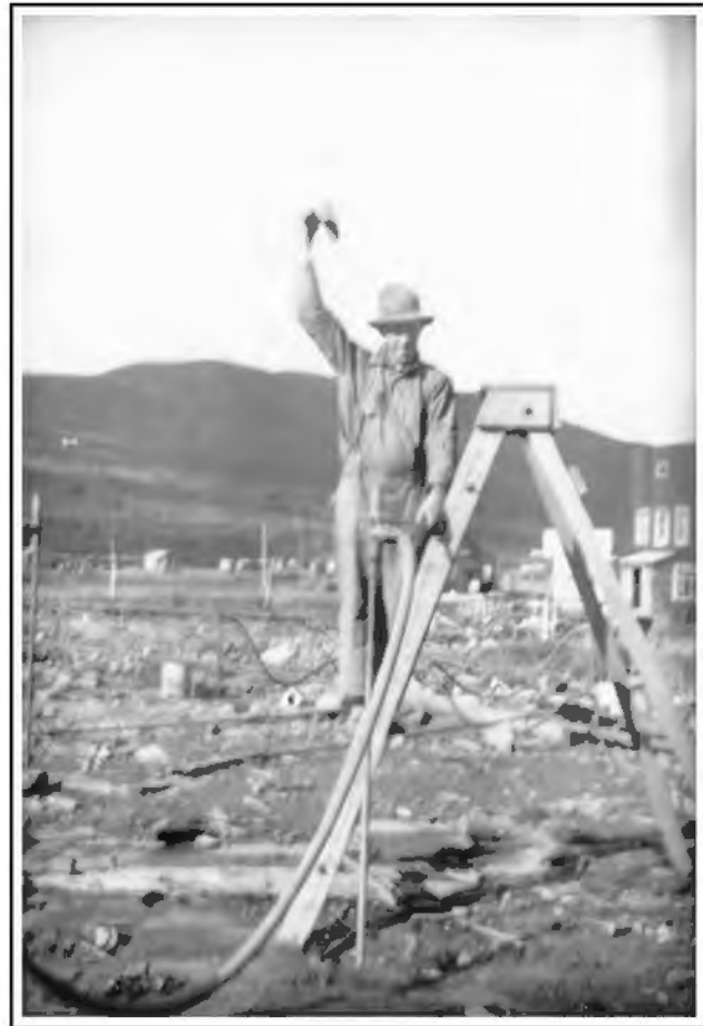
Figure 55. Barnett Photograph #53: An unidentified employee of the Matheson Dredge driving points in Flat.
