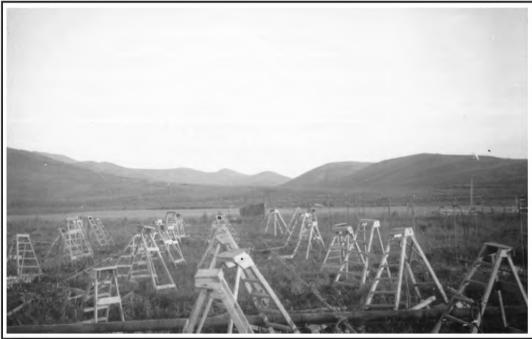
Figure 35. Barnett Photograph #33: Point fields for the Donnelley Dredge, Otter Creek.
