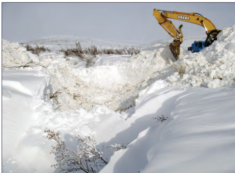
Figure 6. Slotting at crossing AX1 (Seabee Creek). (Photo provided by APC)
