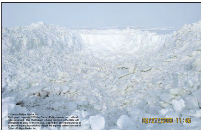
Figure 10. Slotting at crossing CPX3 (Ublutuoch River). (Photo provided by CPAI)
