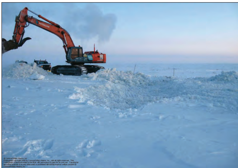
Figure 11. Slotting at crossing CPX4 (unnamed creek). (Photo provided by CPAI)
