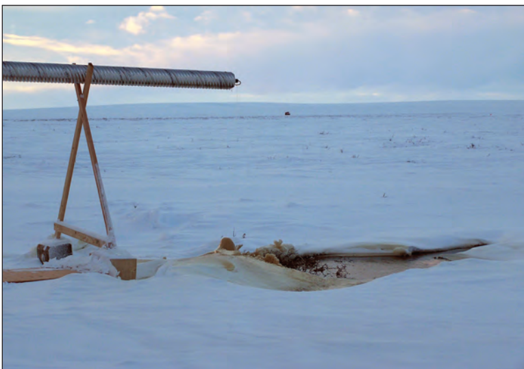
Figure 23. Water discharge from an O&G support camp under the EPA’s NPDES permit.
