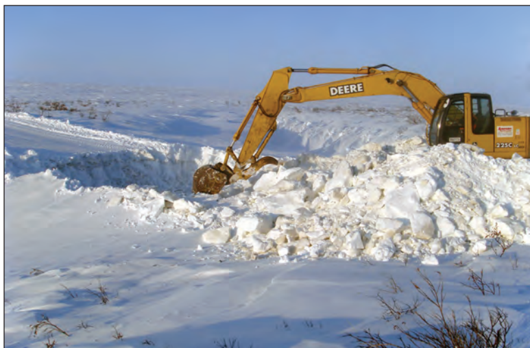
Figure 8. Slotting at crossing AX4 (Prince Creek). (Photo provided by APC)
