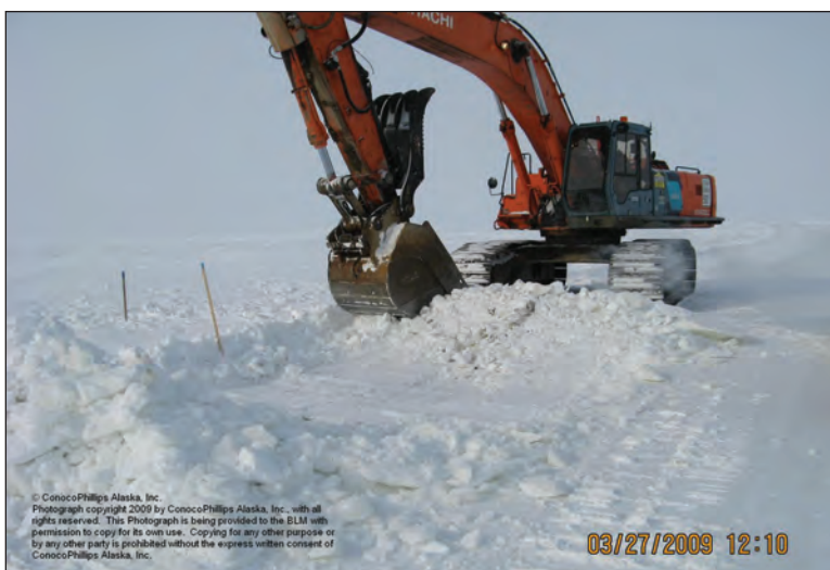
Figure 9. Slotting at crossing CPX2 (unnamed creek). (Photo provided by CPAI)
