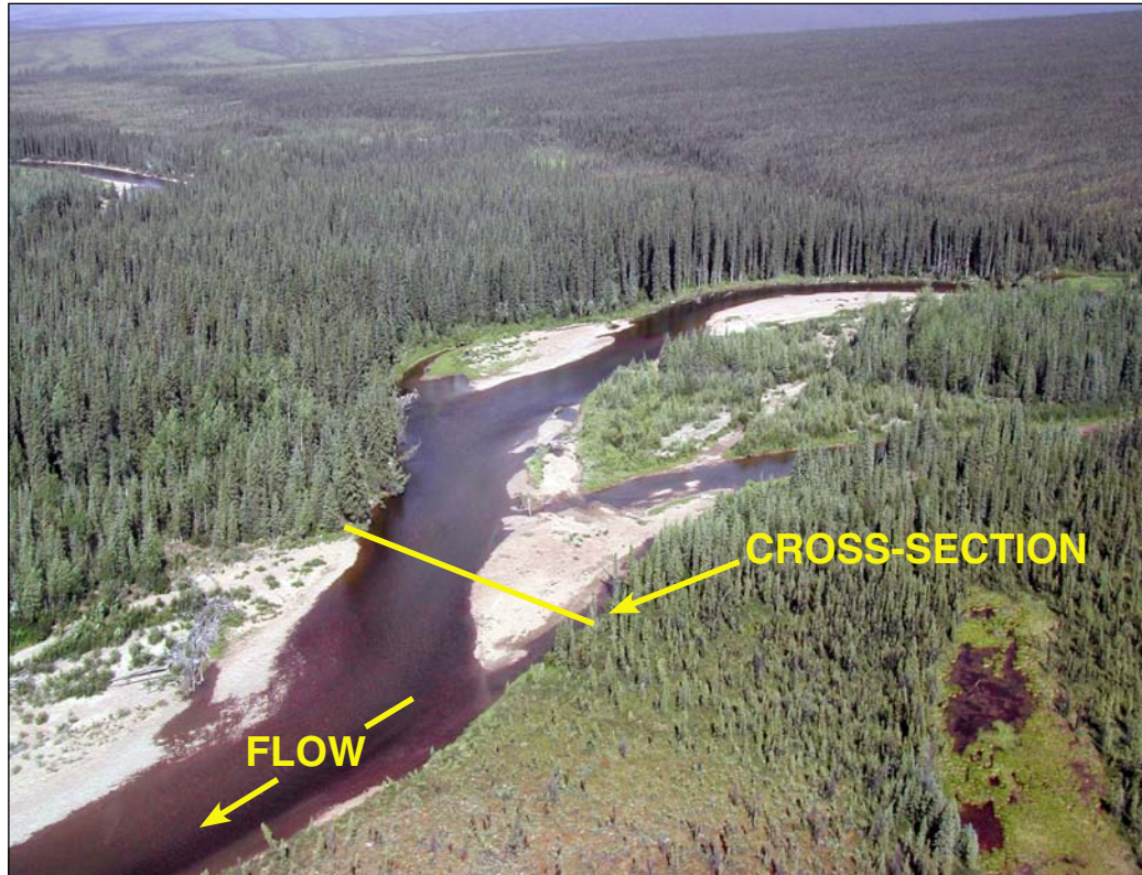
Figure C-3. View of stream channel for Beaver Creek below Nome Creek in July 2003.
