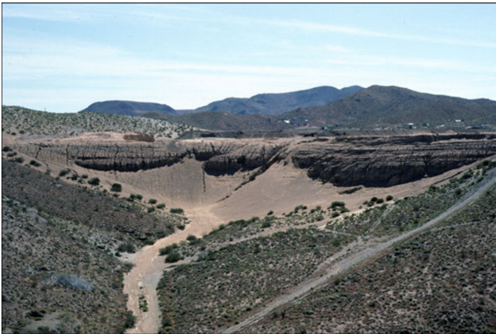
Figure 4.4. Tailings flow, Yellow Aster Mine, Rand Mining District, showing the magnitude of landscape modification, 1993. Note that the tailings blocked the natural drainage but were later breached by erosion (photograph by Karen K. Swope).
