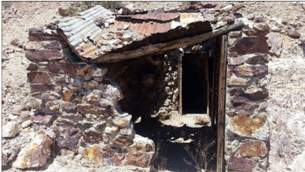
Figure 3.45. Dugout, Copper Strand Mine, San Bernardino County (photograph by Sterling White, BLM).
