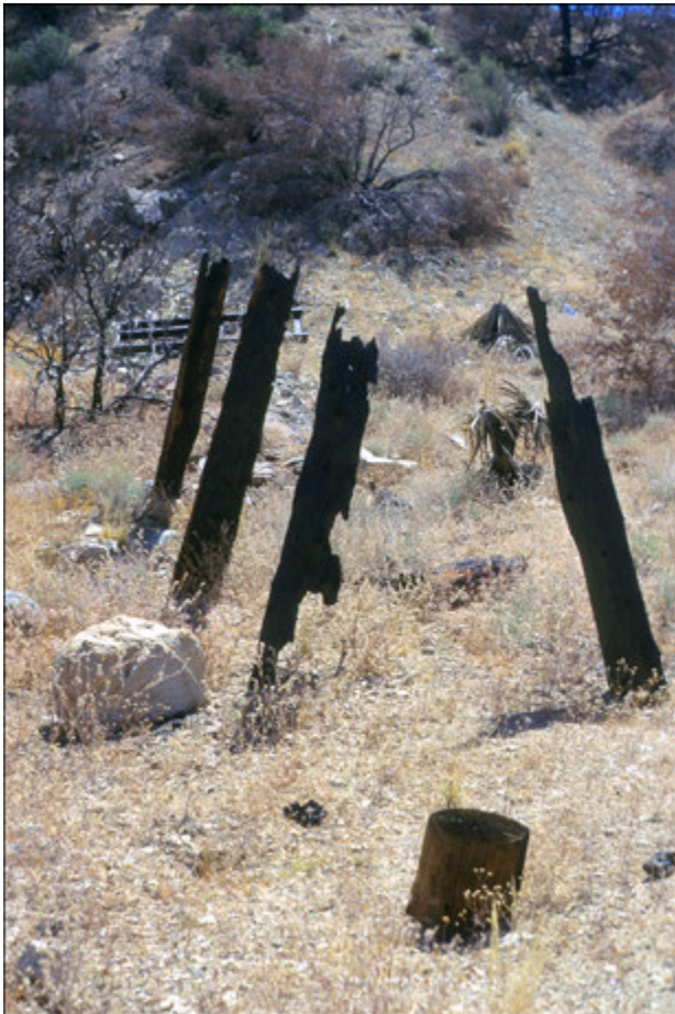
Figure 3.61. Burned ore-car support trestles, Lucky Day No. 1 Mine, Joshua Tree National Park, 1997 (photograph by Karen K. Swope).
