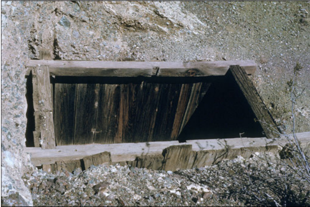
Figure 3.8. Reinforced shaft collar, Red Rock Canyon State Park, 1991 (photograph by Karen K. Swope).
