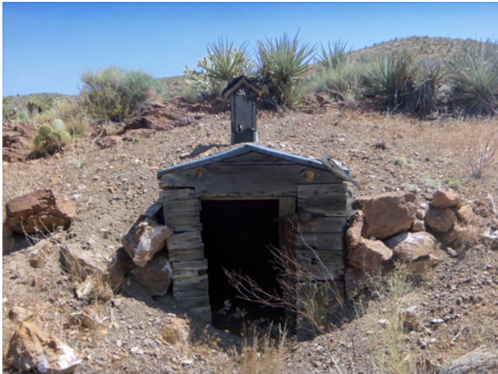
Figure 3.41. Dugout powder-storage facility, Birthday Mine, San Bernardino County, 2011 (photograph courtesy of Statistical Research, Inc.).
