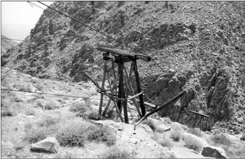
Figure 3.59. Aerial tramway, Beveridge Mining District, Inyo County, 1991 (photograph by Karen K. Swope).
