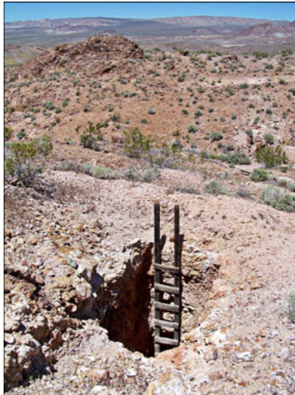
Figure 3.7. Unreinforced shaft collar, Calico Mining District, San Bernardino County (photograph by Sterling White, BLM).
