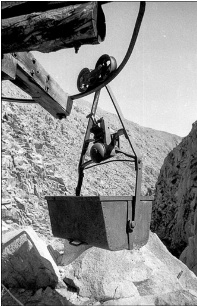
Figure 2.8. Aerial tramway, Beveridge Mining District, Inyo County, 1991 (photograph by Karen K. Swope).
