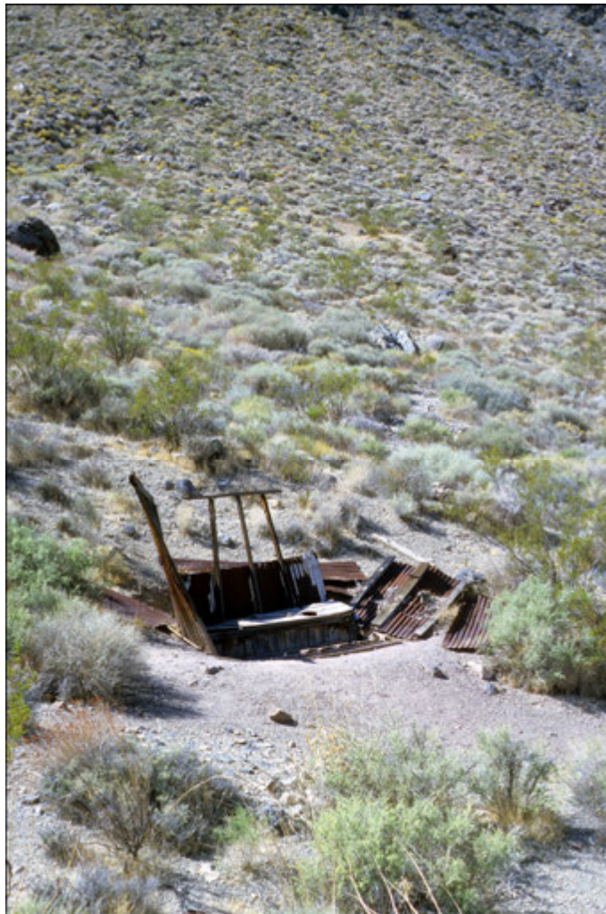
Figure 3.52. Collapsed outhouse, Leadfield, Death Valley National Park, 2000 (photograph by Karen K. Swope).
