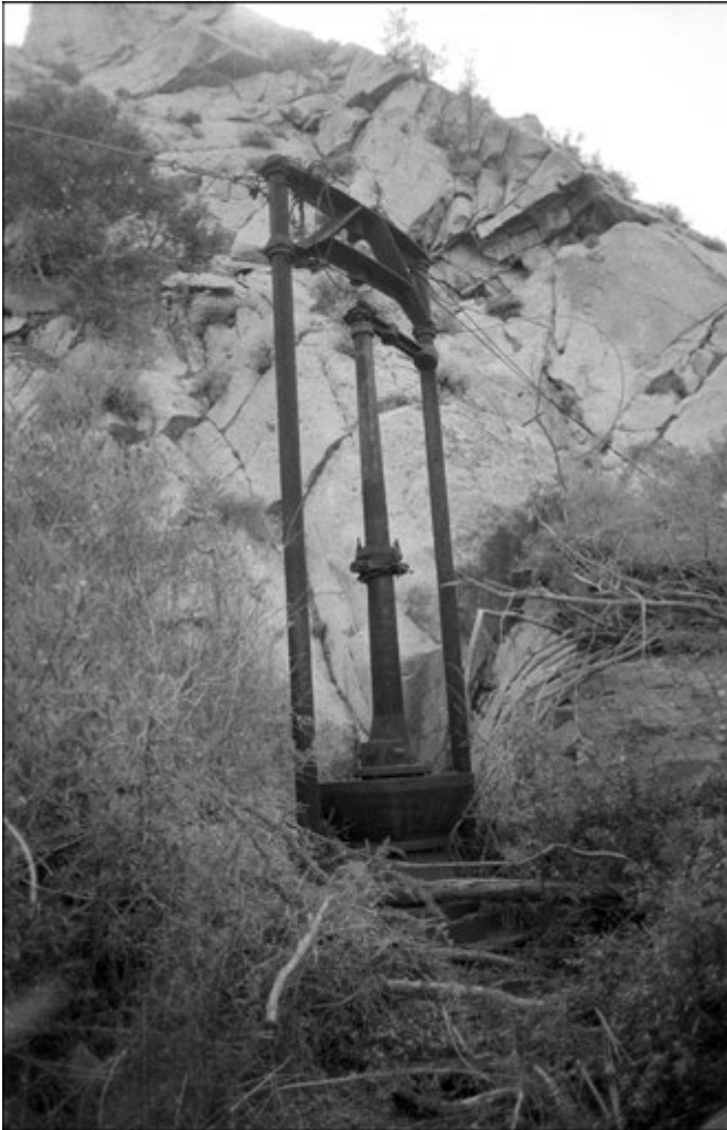
Figure 3.30. Gyratory crusher, Beveridge Mining District, 1991 (photograph by Karen K. Swope).
