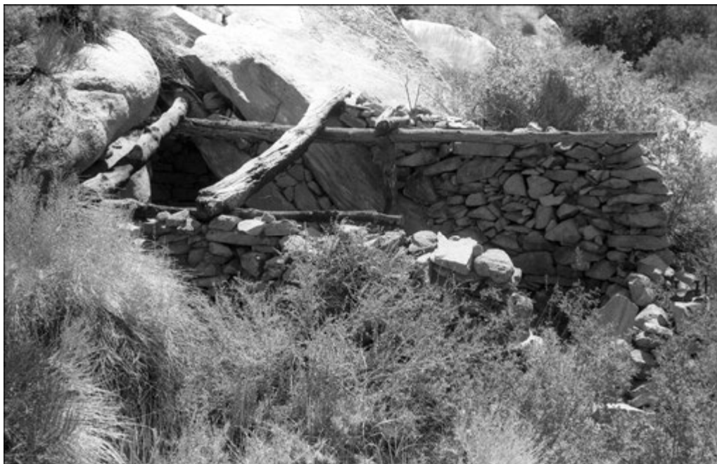
Figure 3.47. Stone dwelling built against a bedrock outcrop, Beveridge Mining District, 1991 (photograph by Karen K. Swope).
