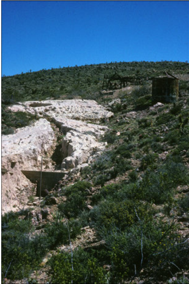
Figure 3.31. Mill tailings, Valley View Mine, San Bernardino County, 1991 (photograph by Karen K. Swope). Note that the tailings overflowed the dam and were later breached by erosion.
