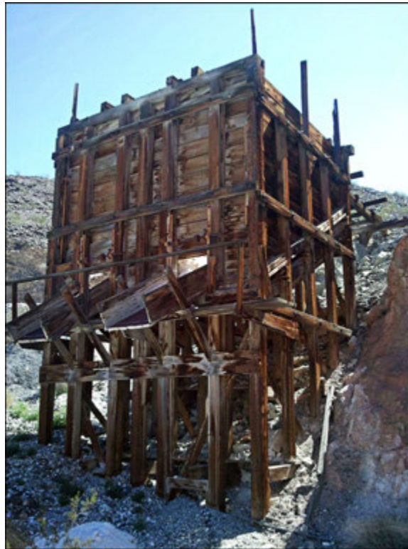
Figure 3.36. Ore bin, Sheep Creek, Avawatz Mountains, San Bernardino County (photograph by Sterling White, BLM).
