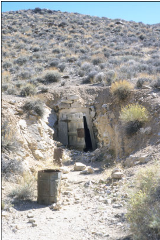
Figure 3.12. Reinforced adit portal, Skidoo, Death Valley National Monument, 1999, (photograph by Karen K. Swope).
