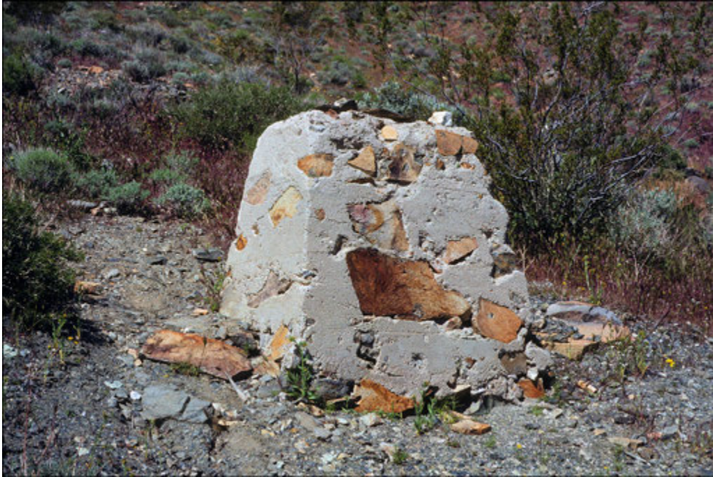
Figure 3.26. Machinery mount, Randsburg Mining District, showing the incorporation of very large rocks in the concrete construction, 1993 (photograph by Karen K. Swope).
