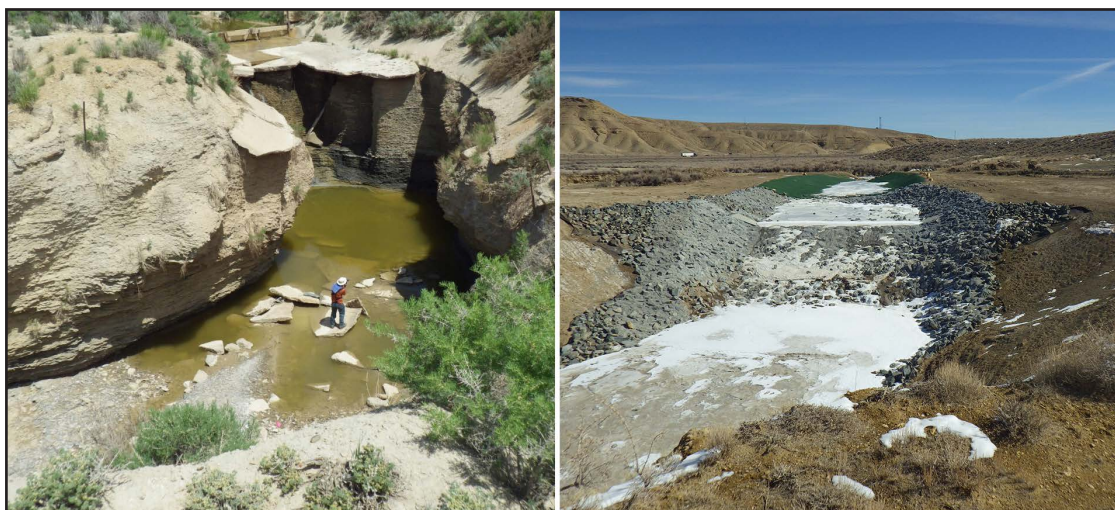
Figure 8. (Left to right) The Pierotto headcut and replacement structure installed in 2016.
