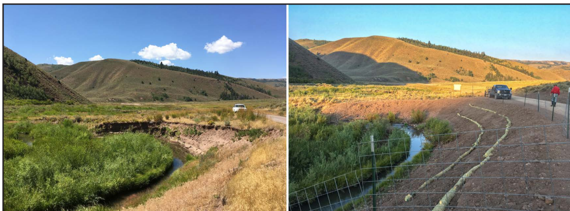
Figure 6. (Left to right) Before and after photos of bank stabilization on Coal Creek
