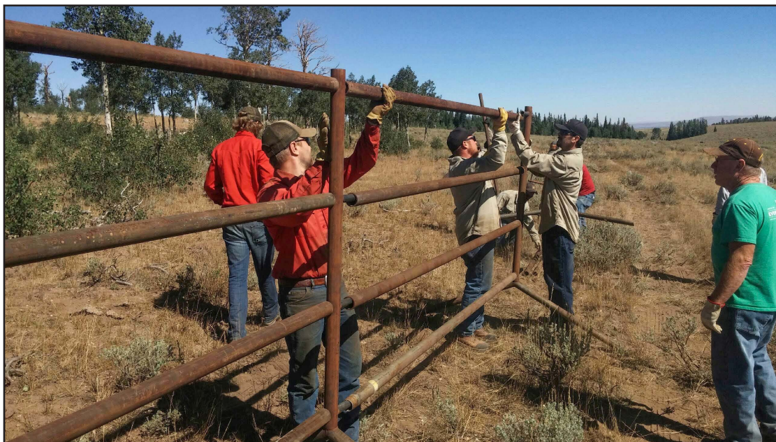
Figure 4. Project members work to install steel jack fence near Little Mountain aspen stands to exclude ungulate use and promote unimpeded vertical regeneration.
