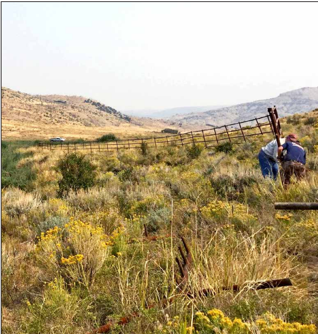
Figure 14. Steel Jack fence installation along Trout Creek to protect riparian corridor. Photo courtesy of Trout Unlimited.
