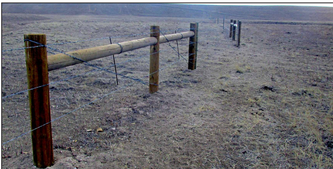
Figure 21. A completed section of wildlife friendly fence. Photo courtesy of the Medicine Bow Conservation District.
