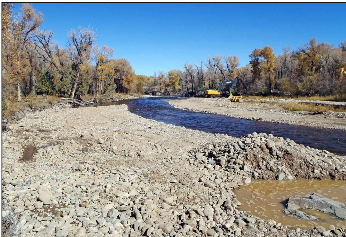
Figure 13. Constructing a narrower and deeper channel at the Encampment River - Riverside Phase I Restoration. Photo credit WGFD.
