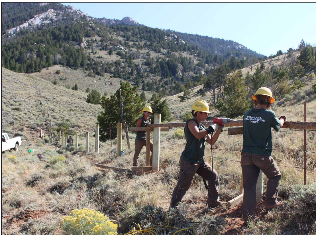
Figure 2. Montana Conservation Corps crew modifying old barbed and mesh wire fence to wood post, rail-top and wire fence on Ferris Mountain. Photo credit BLM.
