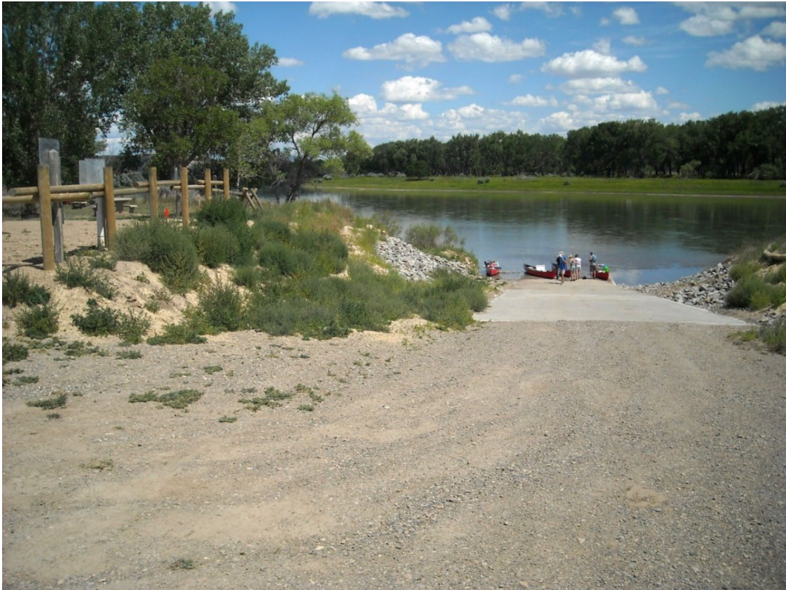
Figure 1: The new boat ramp at Coal Banks recreation area
