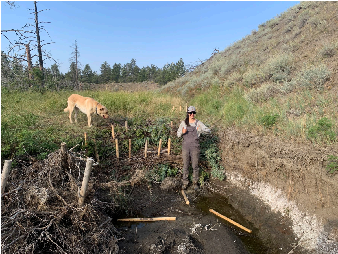
Figure 4: Volunteer from the National Wildlife Federation constructing a beaver dam analog within Reed Coulee
