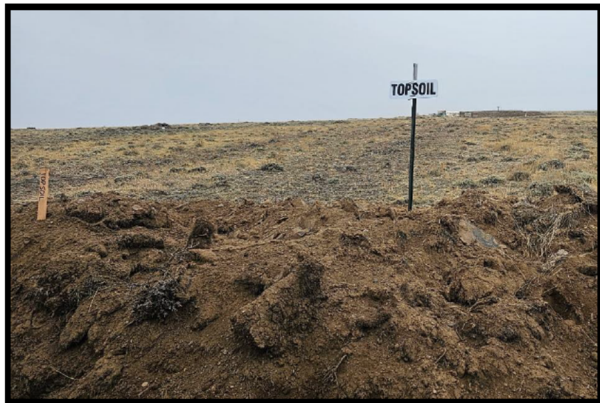
Figure 7: Photograph of a topsoil stockpile at a drill site with signage.
