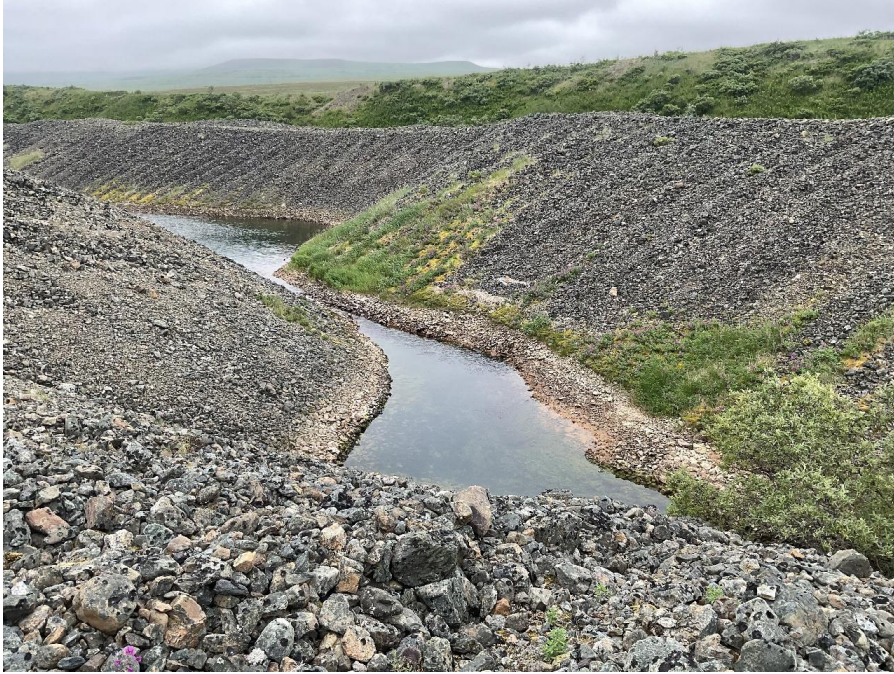
Photograph 24. Example of a ponded section in the tailings that is adjacent to a dry stream section and shows clear signs of stream flow emerging from the upstream end of the ponded area and exiting at the downstream end near where the mainstem Salmon River begins surface flows again.
