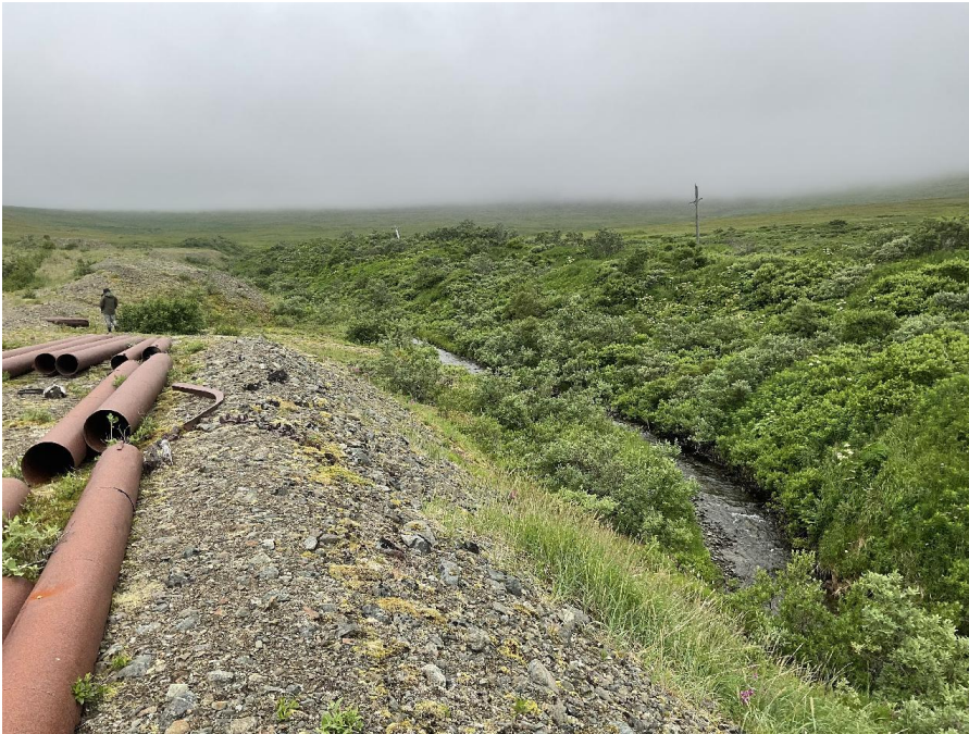
Photograph 11. Upstream view of Platinum Creek valley where tailing piles confine the stream and limit floodplain development.
