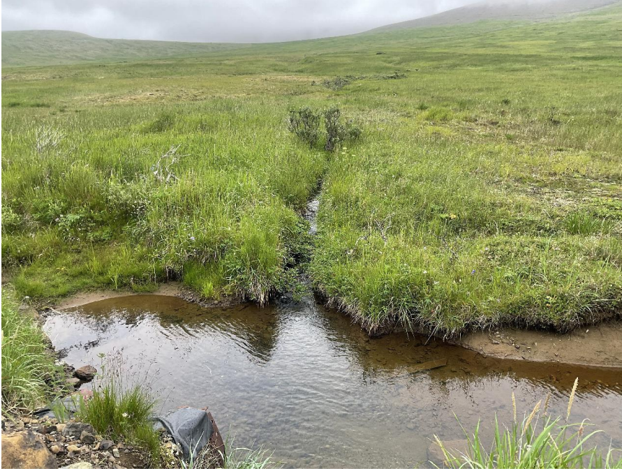
Photograph 6. Boulder Creek where the channel is ponded upstream of the road crossing, likely indicating it may be undersized.
