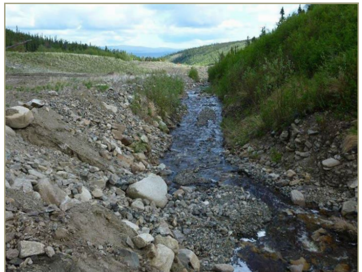
Photo 41. This poorly constructed stream has little to no floodplain connectivity because it likely will not overtop and spread water across its potential floodplain on the left. From BLM's " Stream Reclamation Basics ."
