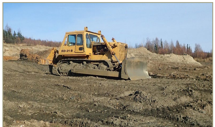
Photo 16. Dozer, Hot Springs Mining District Alaska 2021 (DNR).
