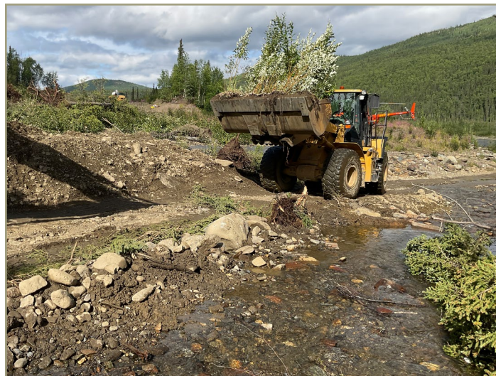
Photo 36. Wheel-loader moving an intact block of soil and vegetation (vegetation mat) from a source (donor) site to an area being reclaimed. This creates “instant” vegetation. From BLM’s “Stream Reclamation Basics.”
