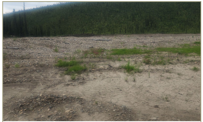
Photo 38. Photo showing floodplain with varying terrain, including a small conveyance swale leading to a reclaimed pond. Seen in the picture is a micro-depression located in the swale with sediment deposition occurring during highwater events. Since this photo was taken (July 2023), additional organics were speared on site to encourage faster revegetation rates - the area is now (August 2025) mostly revegetated (USACE).
