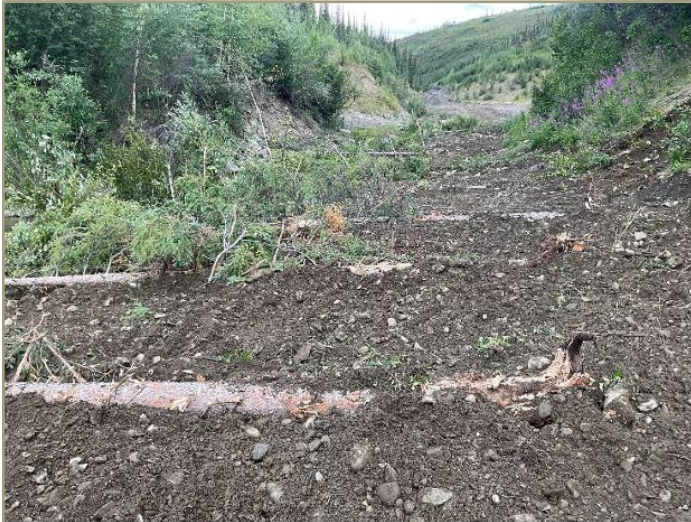
Photo 42. Spruce logs and vegetation transplant mats used to minimize floodplain erosion until vegetation is fully reestablished. From BLM's "Stream Reclamation Basics."
