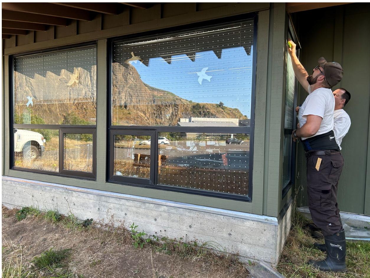
BLM maintenance staff install window film that leaves a white-dot pattern designed to minimize bird-window collisions
