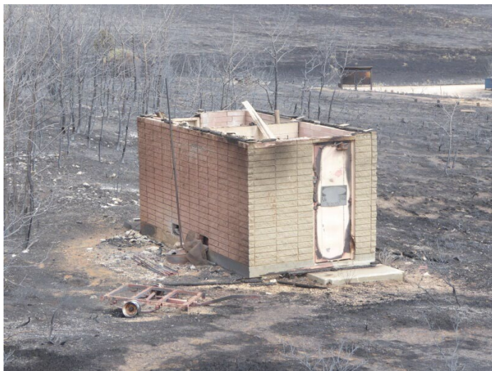
Wildhorse burned vault toilet
