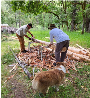
BLM Staff Peeling Logs for Cabin Renovation
