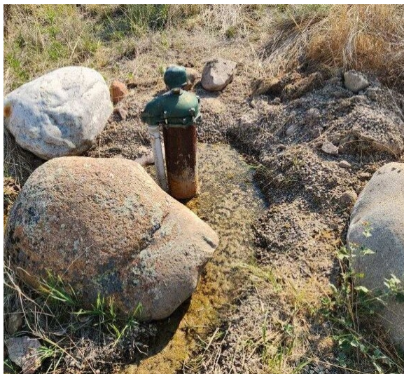
Photo of leaking wellhead at Cottonwood Campground
