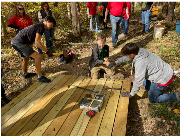
Eagle Scout building a new puncheon bridge
