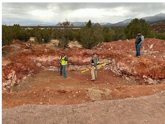
Digging a hole for a new vault toilet
