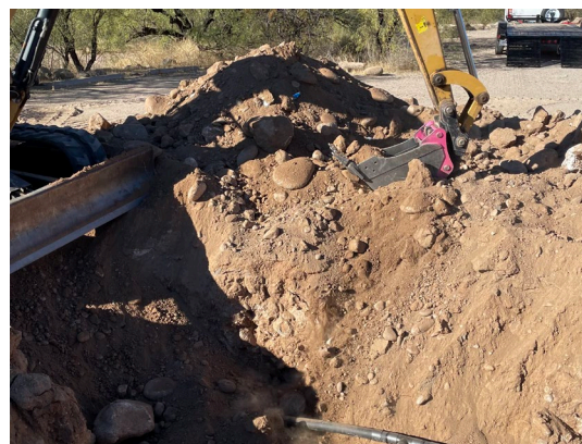
Excavator Backfills Waterline at Burro Creek
