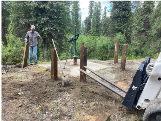
Installation of parking barriers
