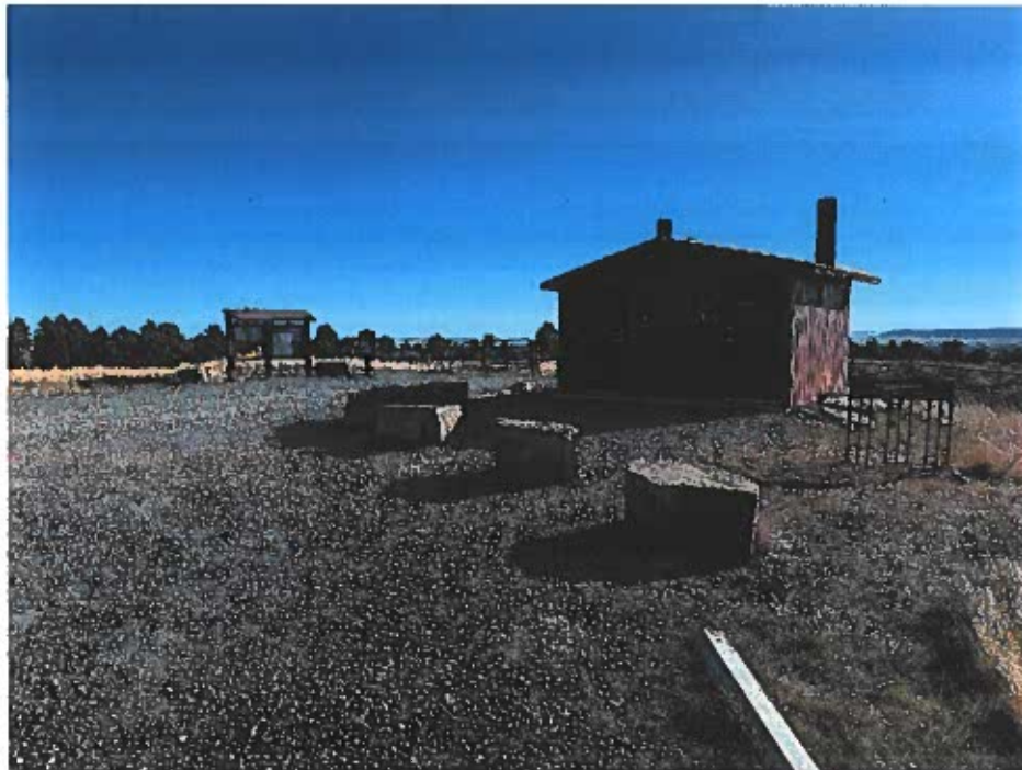
Photo 9 – Vault toilet and information kiosk at trailhead.
