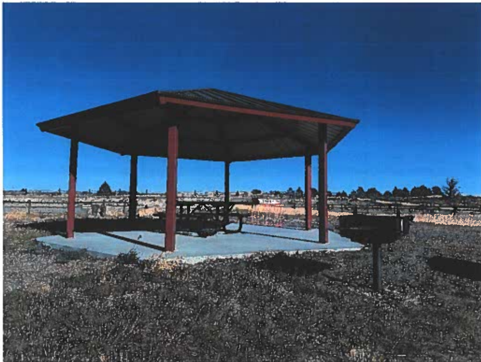
Photo 8 – Shade structure, accessible picnic table, and grill at trailhead.
