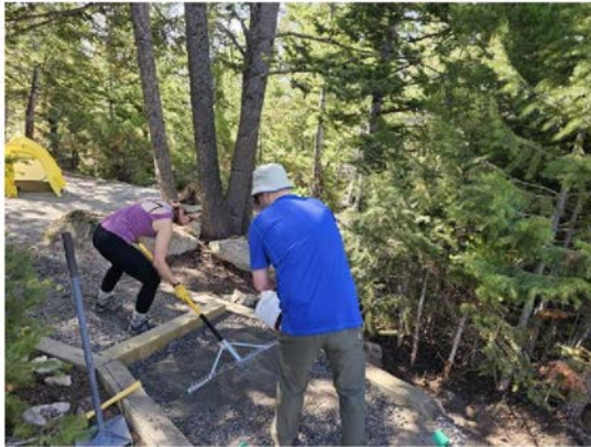
AHS volunteers help fix damage to a campsite
