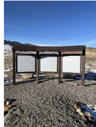
A 3-Panel Kiosk is installed at Outlaw Trailhead
