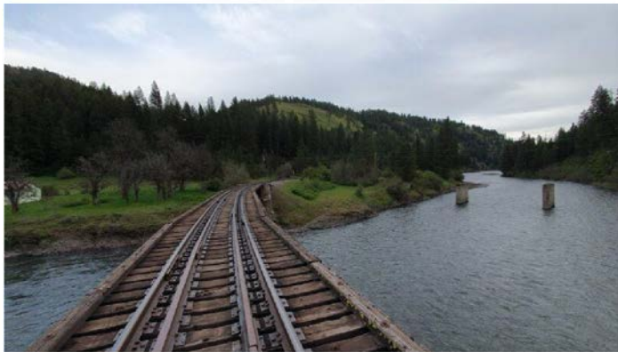
Bridge over Grande Ronde
