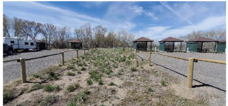
Fencing project at Egin Lakes Campground
