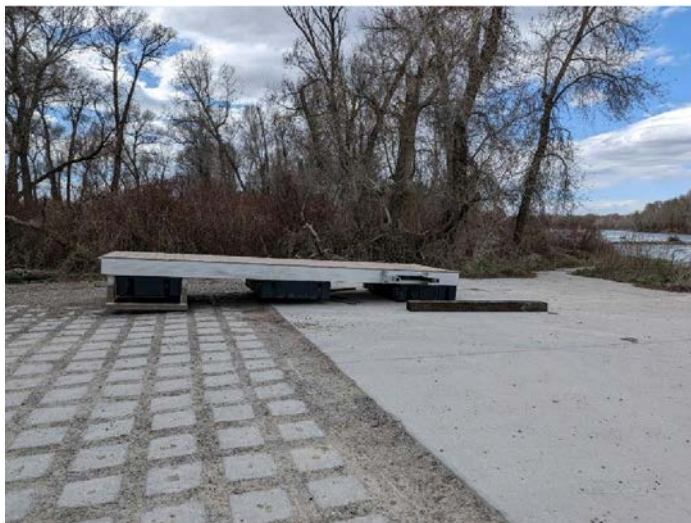
Dock improvements at Lorenzo Boat Access
